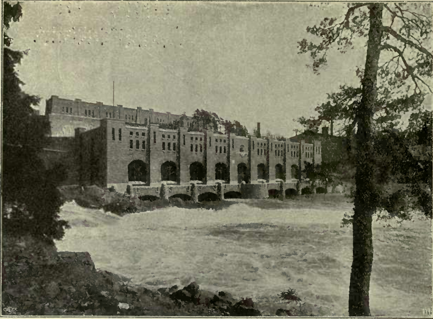
TROLLHÄTTAN POWER STATION
